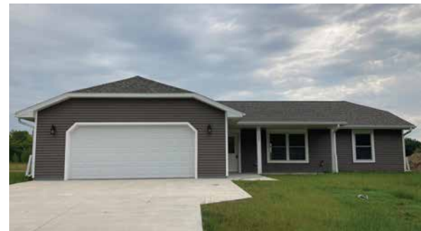
CLT in Miltona, Minnesota
